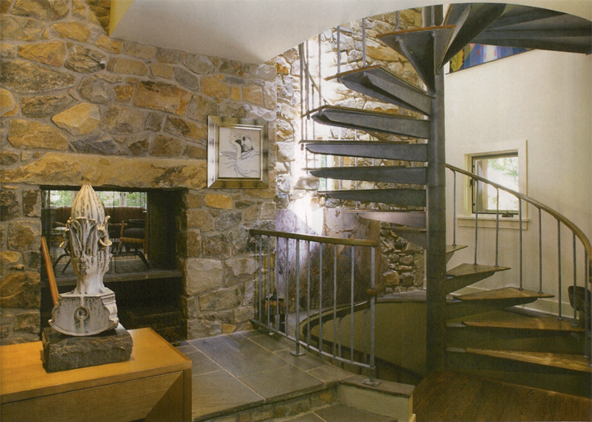
ABOVE: THE WEIGHTLESS LOOK OF THE COMMERCIAL SPIRAL STAIR IS OFFSET BY THE STURDY STONE WALLS AND FLAGSTONE FLOOR.
